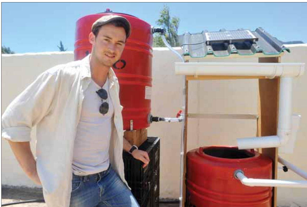
Water-borne: Benjamin Biggs (in picture) and Carl Jacobs developed and tested an application that uses a solar-powered pump to facilitate the re-use of grey and/or rainwater at domestic household level.
