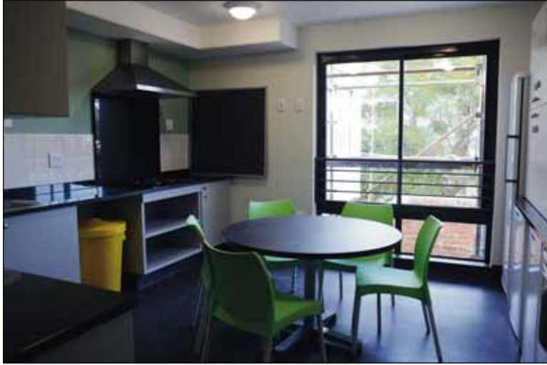
Making room: One of the completed kitchens in the Obz Square residence, currently under construction.
