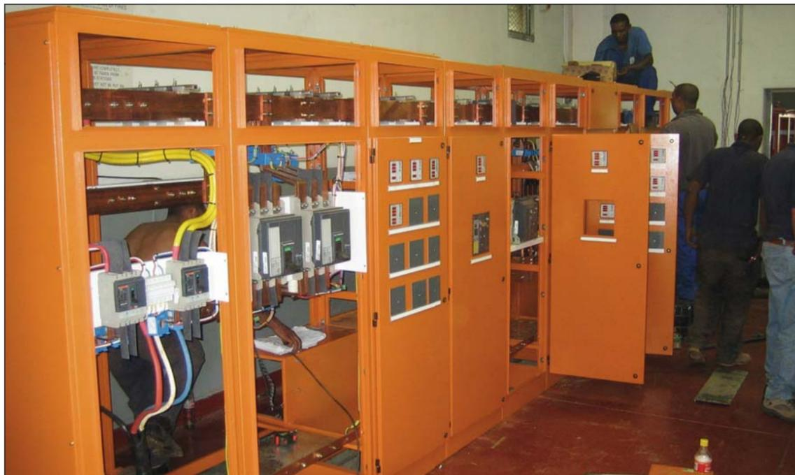
Wired: An upgrade to the Jameson substation was recently completed by Properties and Services. Pictured here is a team of contractors installing the new main 400V distribution board.
